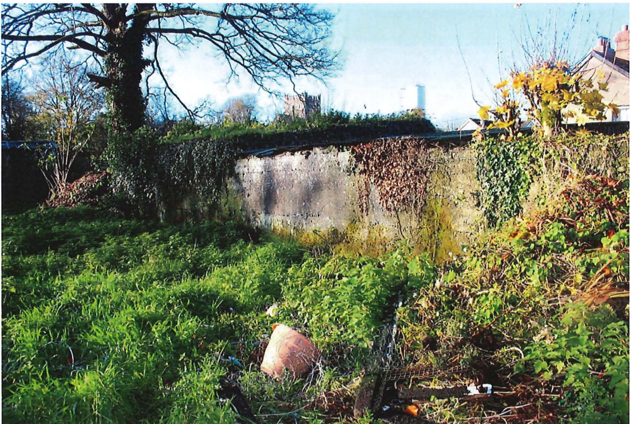
Fig. 22 – View southwest – C. 1900 pair of red-brick semi-detached houses concrete boundary wall.
