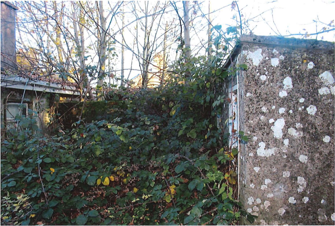
Fig. 40 – View north, mid-20 th kitchen extension (room 1-03) to the west and outbuilding (room 1-07) to the west.
