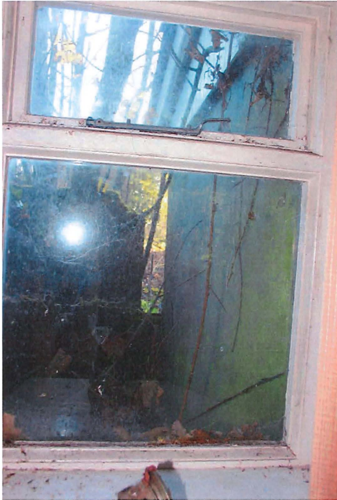
Fig. 28— Room 2-02, looking east. Non-original timber window.
