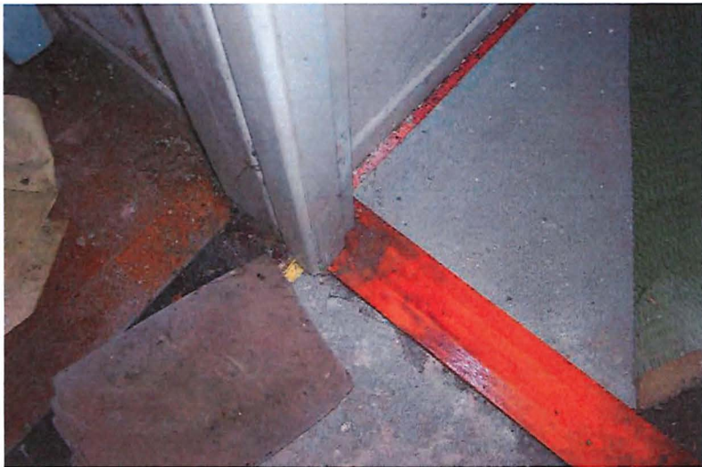
Fig. 46 – Rooms 3-02 & 3-03, concrete floor slab.
