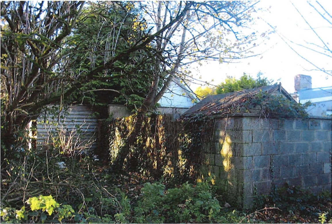
Fig. 17 – View south – Concrete block boundary wall and corrugated fence.
