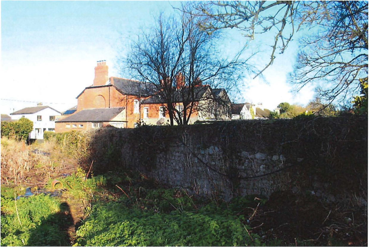
Fig. 19 – View northwest –End-19 th century rubble stone wall section.
