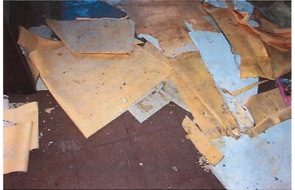
Fig. 41 – Room 2-06, tiled floor finish.
