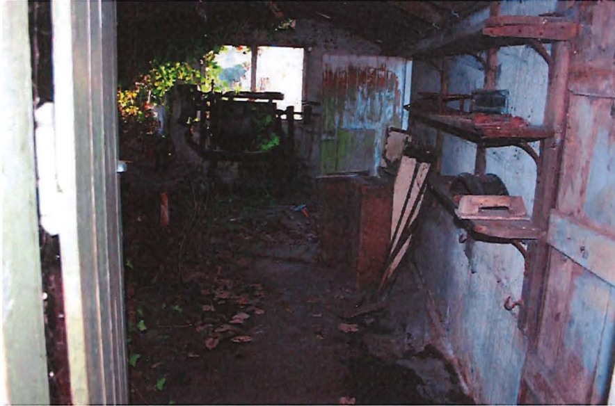
Fig. 32– Room 2-05, looking east, first-half of mid-20 th century cobbler workshop. Concrete slabs and concrete blockwork walls.
