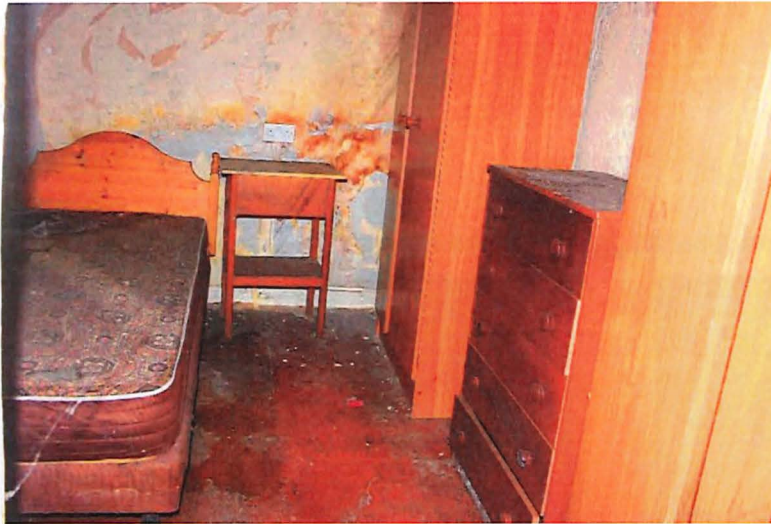
Fig. 4 – Room 1-02, looking south. Linoleum floor finish and wall paper finish.
