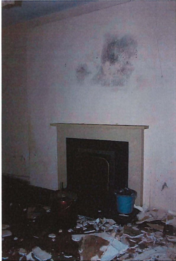
Fig. 12 – Room 1-04, looking north. Non-original fireplace.
