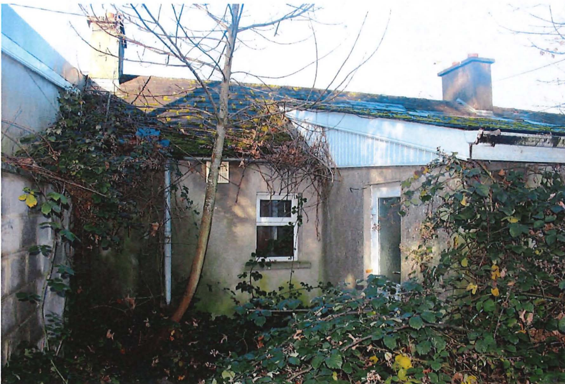
Fig. 39 – Cottages, east elevation, south section and mid-20 th kitchen extension.
