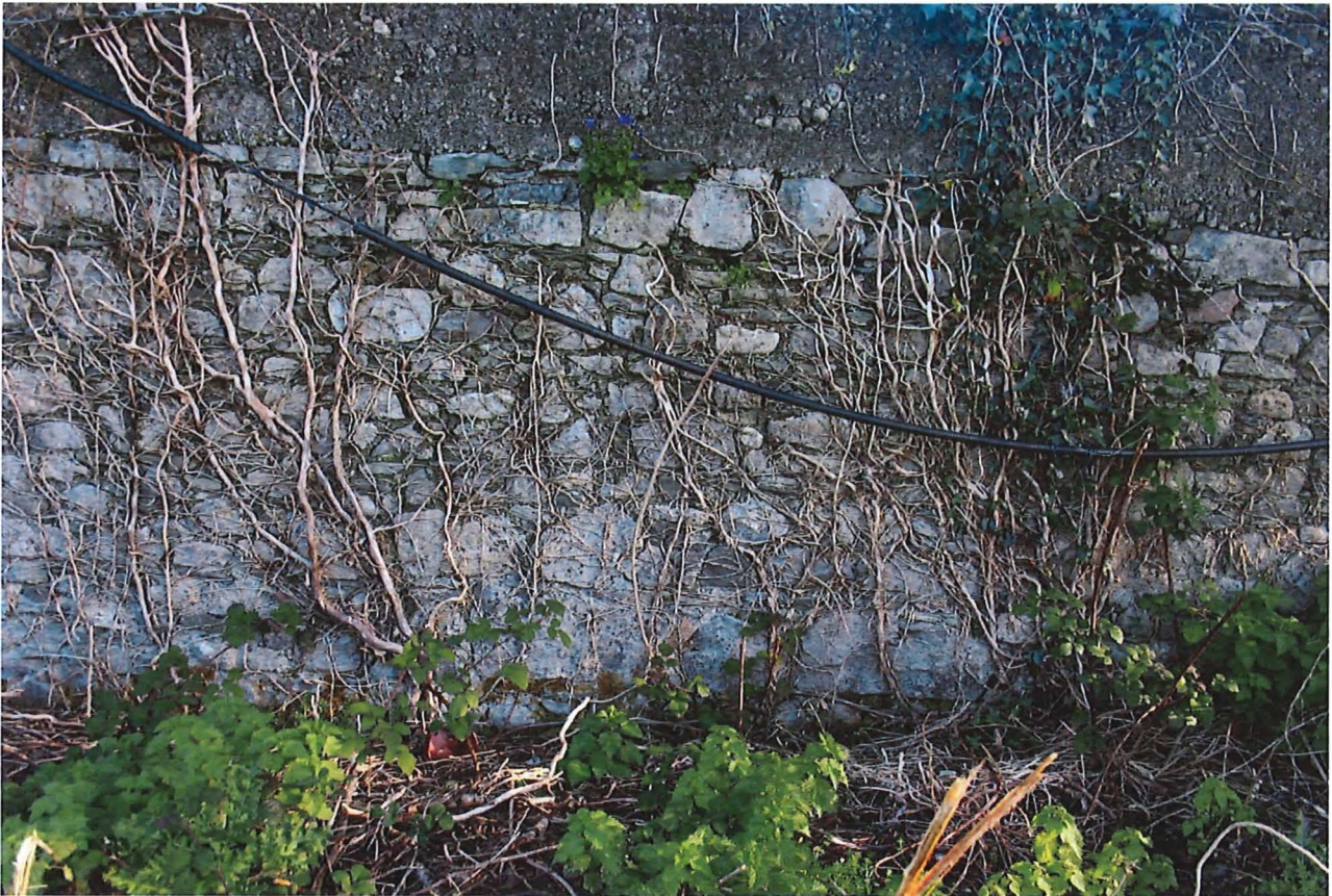
Fig. 30 – View north. End-19 th century rubble stone wall section.
