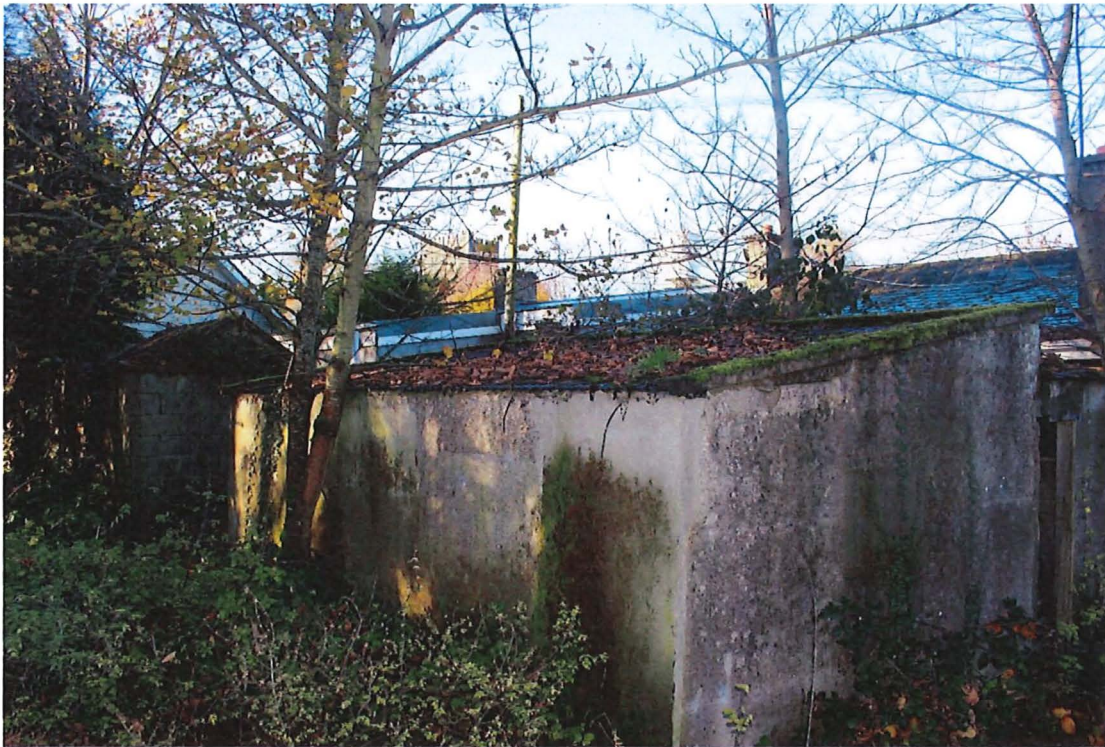
Fig. 37 – Mid-20 th outbuilding, rooms 1-06 and 1-07
