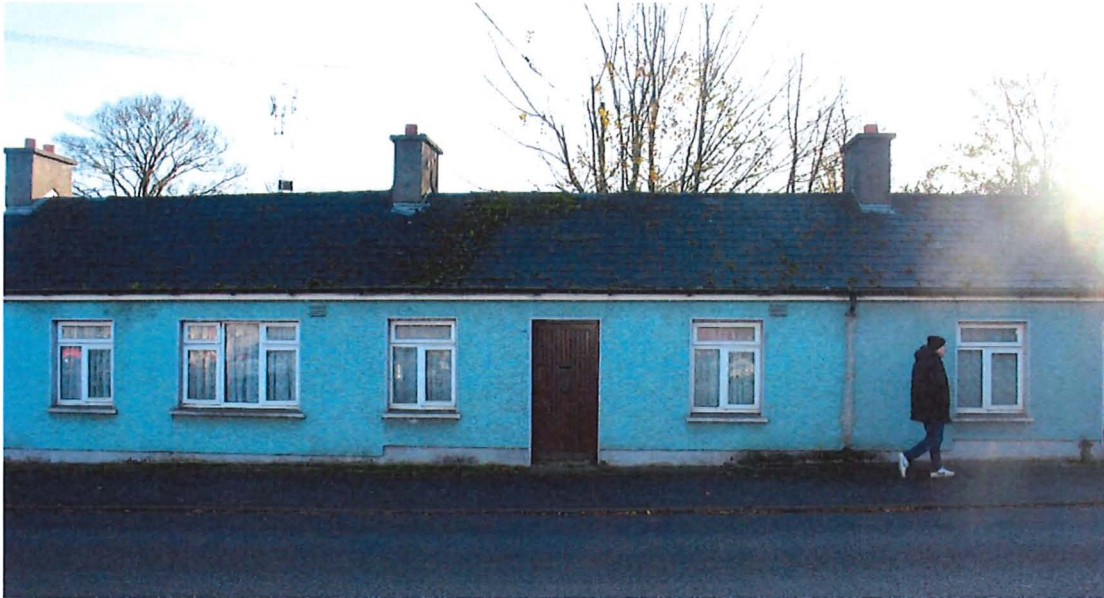
Fig. 9 – View east on Station Road –Subject cottages, central section.
