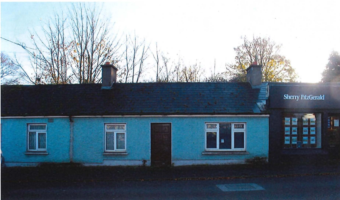
Fig. 8 – View east on Station Road –Subject cottages, south section.
