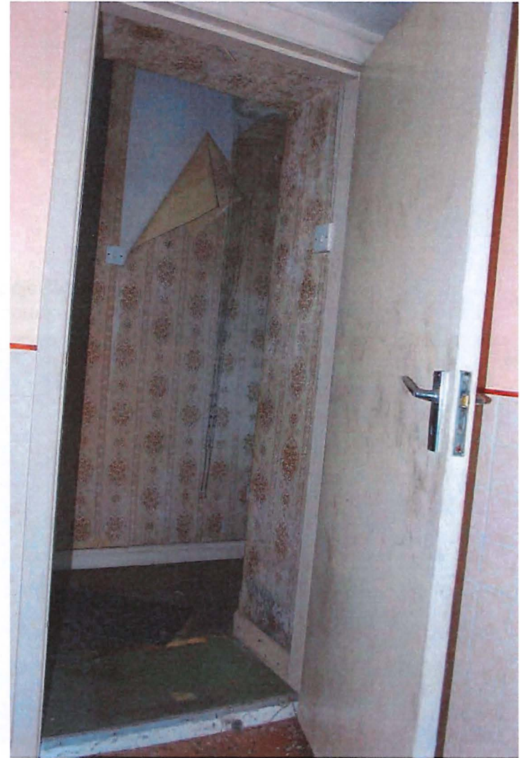
Fig. 31– Room 2-03, looking west to room 2-02, non-original timber door.
