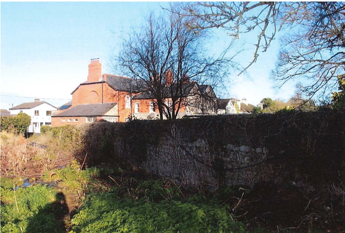
Figure 12: View north. End 19 th -century rubble stone wall section.
