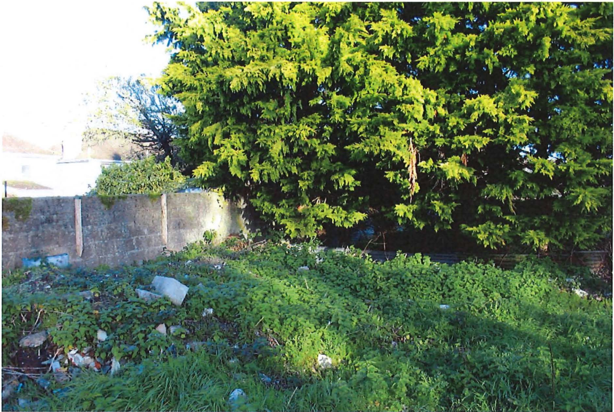
Fig. 23 – View northwest – Concrete blocks boundary wall and corrugated fence.
