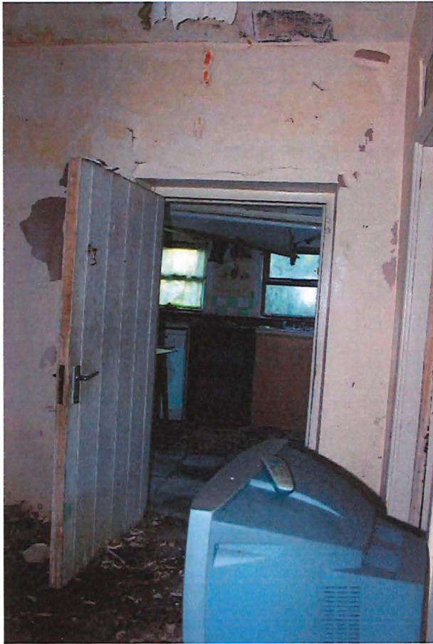
Fig. 9 – Room 1-04, looking east. Non-original timber door.
