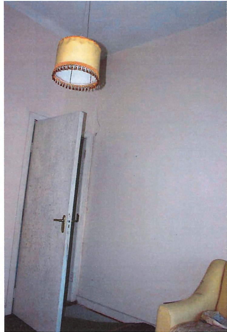
Fig. 52– Room 3-04, looking southeast. Non-original timber door.
