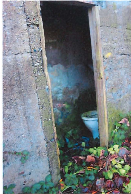
Fig. 18 – Room 1-06, mid-20 th century outbuilding.
