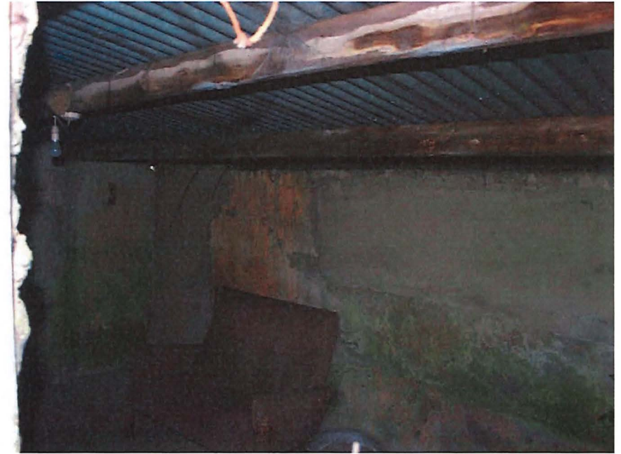
Fig. 19 – Room 1-07, mid-20 th century outbuilding.
