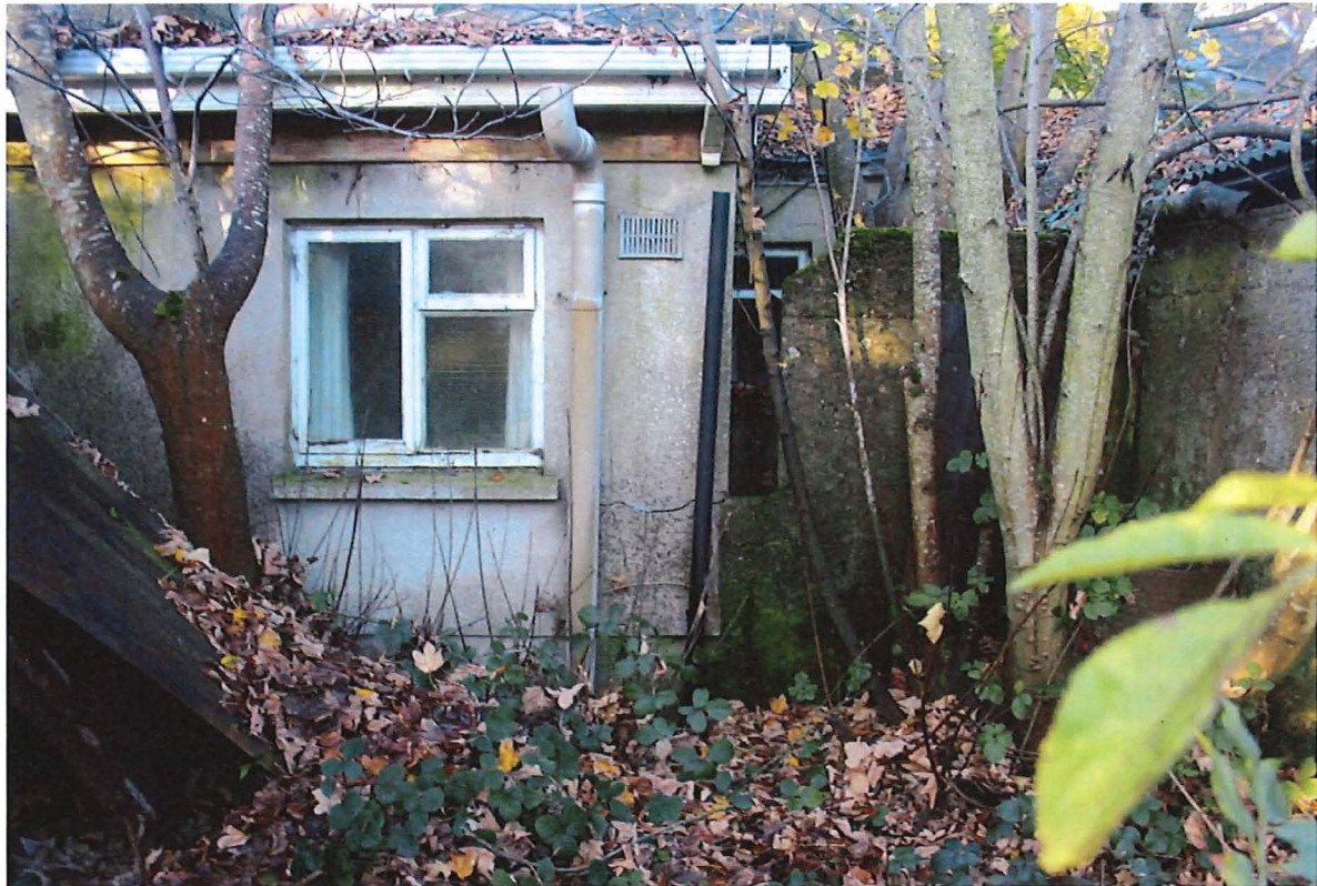
Fig. 34 – Looking at the mid-20 th century bathroom extension, rooms 2-03, 2-04.
