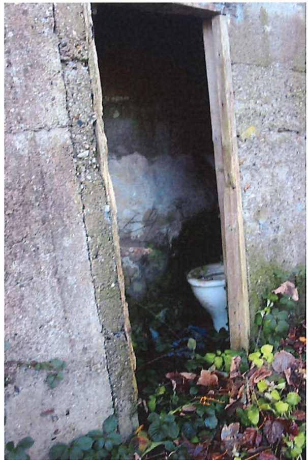
Fig. 33 – Mid-20 th century outbuilding extension, room 1-06.
