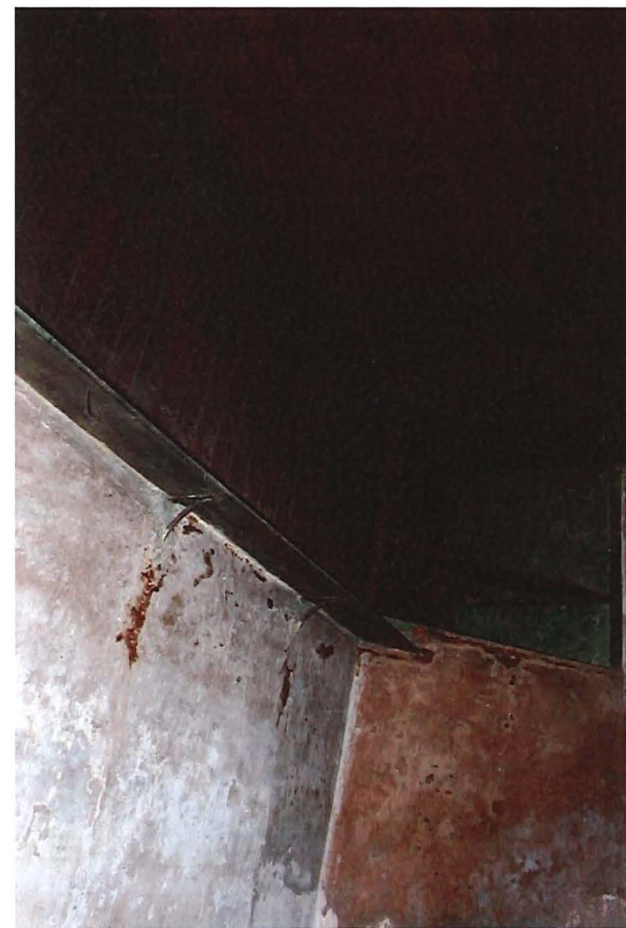
Fig. 3 – Room 1-01, top section of chimney breast was removed.
