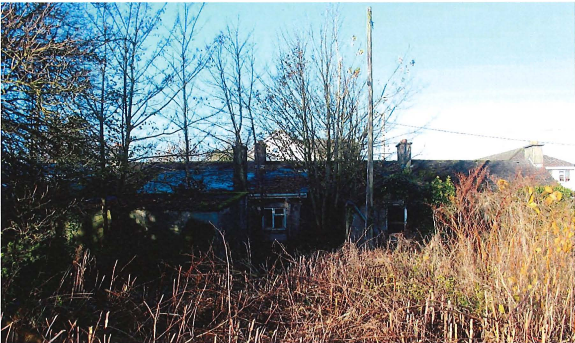
Fig. 41 – East elevation, subject cottages.
