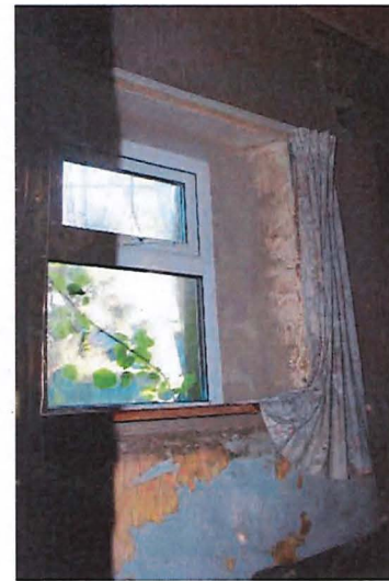
Fig. 7 – Room 1-02, looking east. uPVC window.
