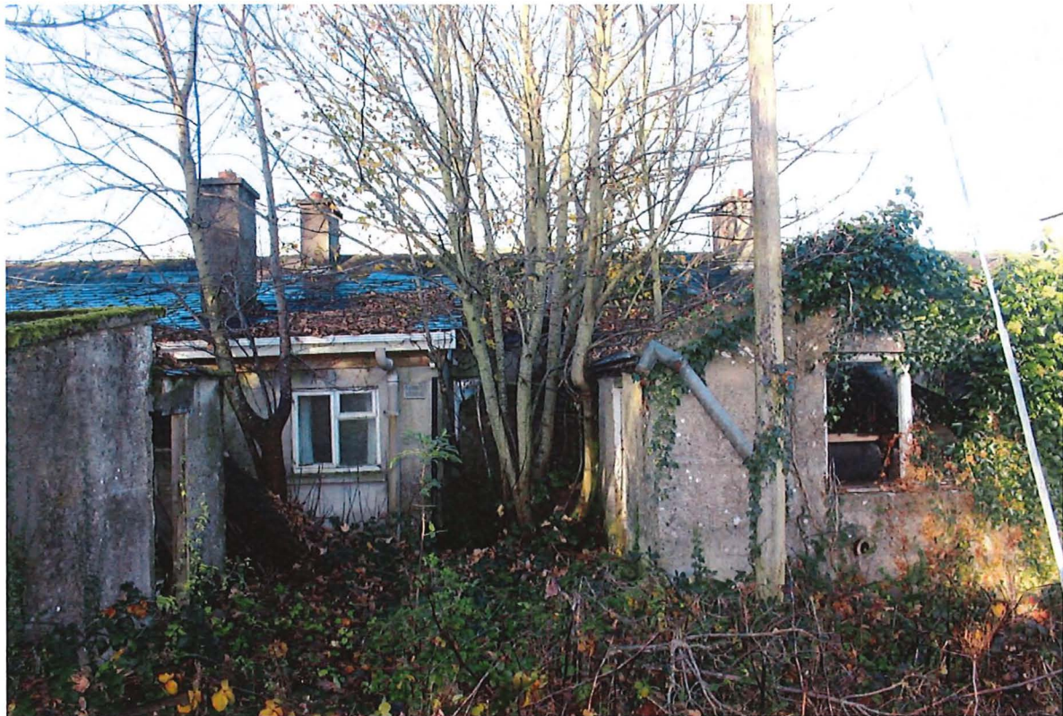
Fig. 35 – Mid-20 th century bathroom extension, rooms 2-03, 2-04 and first half mid-20 th cobbler's workshop, room 2-05 with outbuildings, rooms 1-06 and 1-07.
