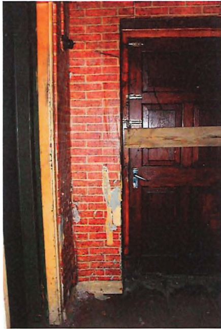
Fig. 17 – Room 1-05, non-original timber entrance door.
