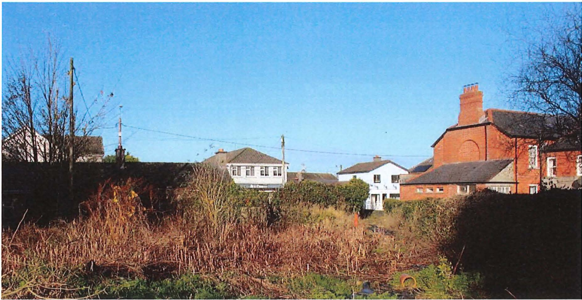
Figure 19: Rear of cottages with modern extension to the north.
